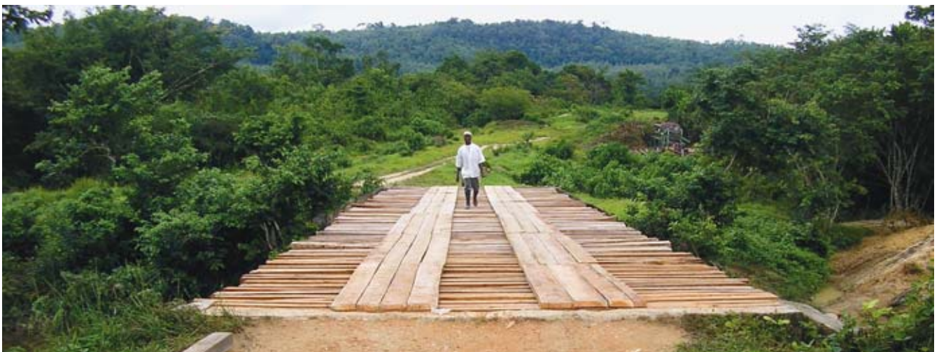
Butulu Bridge Rehabilitation
