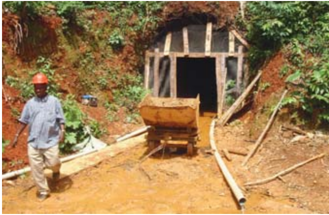
Rehabilitation of the old working adit
