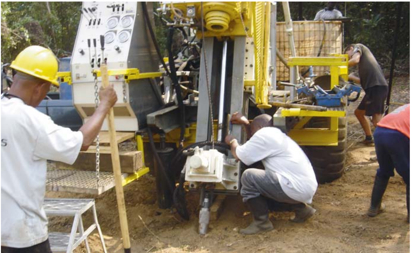
Drill rig set up at NLGM
